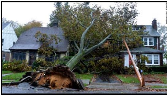
Downed trees in Garden City, NY after Hurricane Sandy. Photo Credit: CNN.
