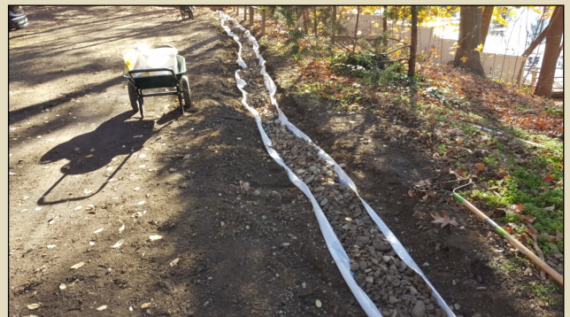
Installing the drainage pipe. Cedarmere Preserve
