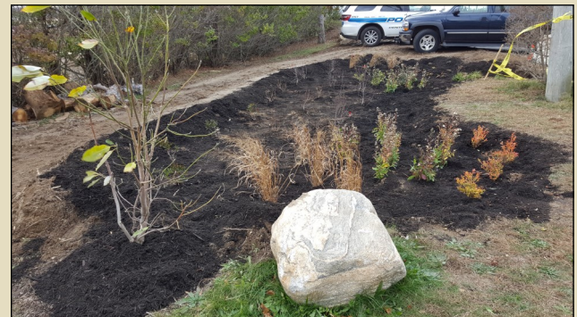
A completed raingarden. Centre Island.
