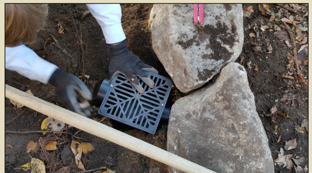
Installing a catch basin. Cedarmere Preserve
